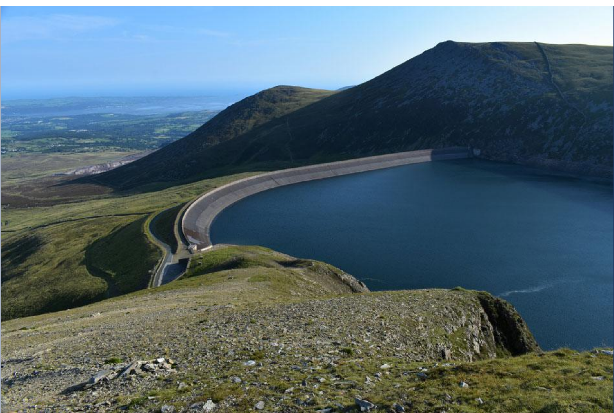
This is Marchlyn Mawr dam in Wales which is similar to the dams proposed at Earba
