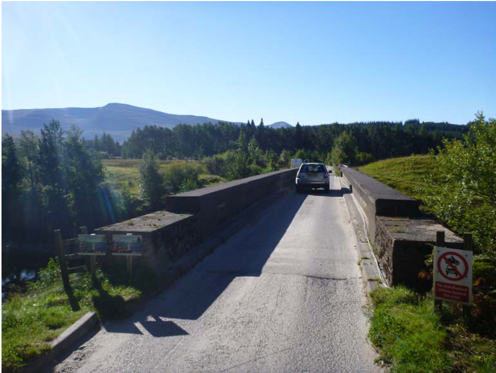
L01 - Entrance to Moy Bridge from the A86
