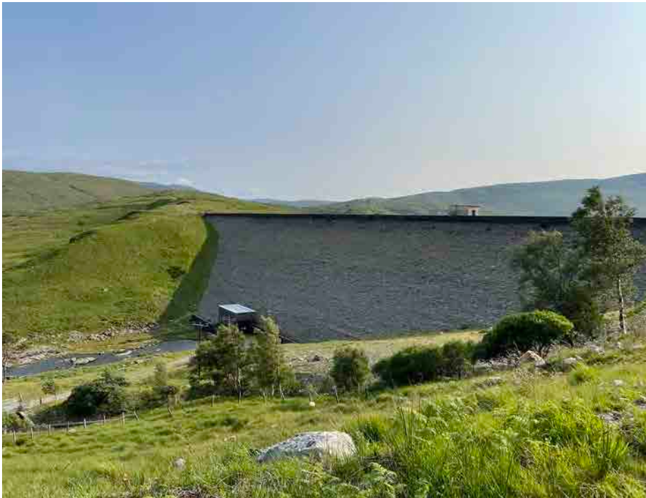
Figure 09 Quoich Dam rockfill elevation with valve house roof & intake protruding above the dam
