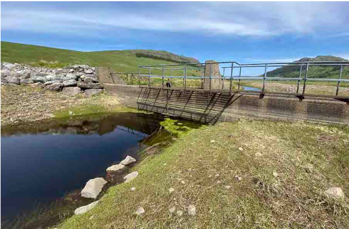
Figure 13 The upstream view of the structure that controls water flow between the two lochs
