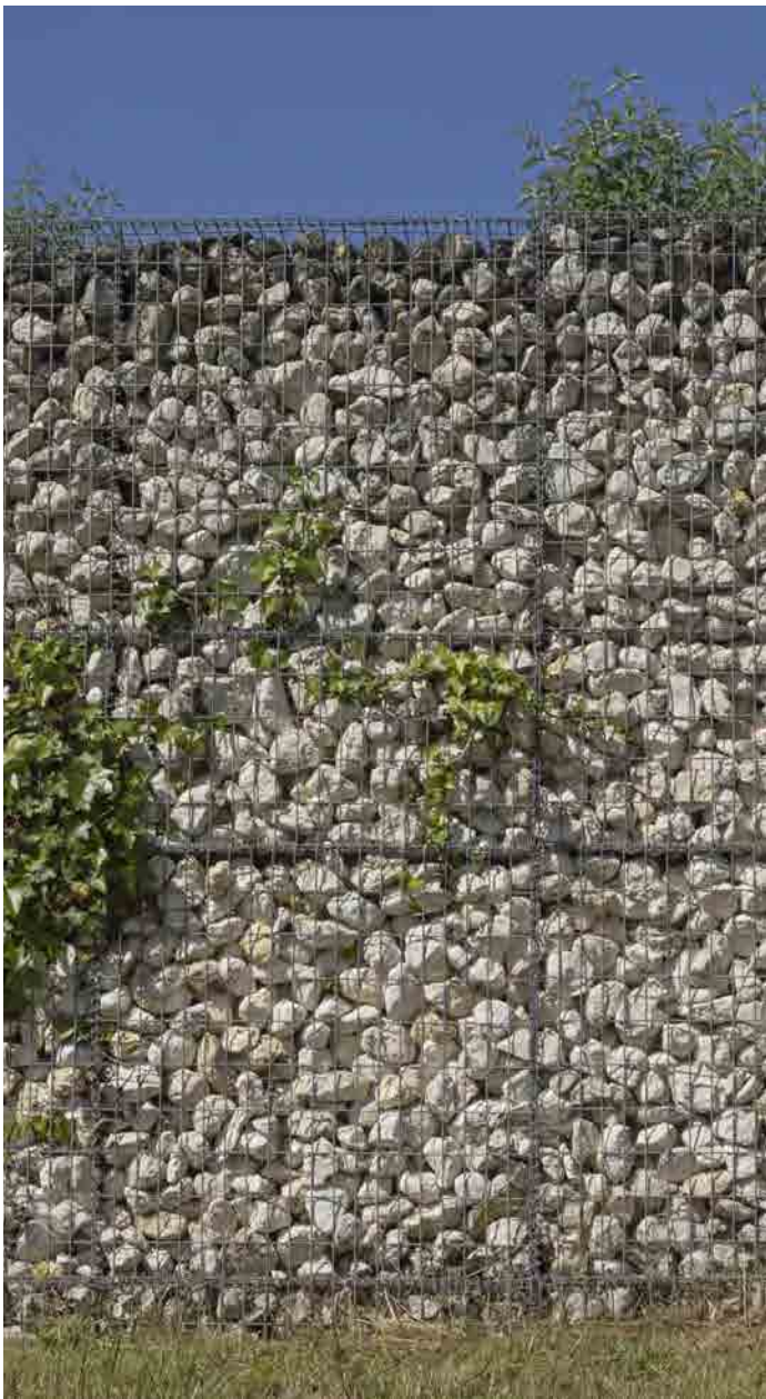
01 - variation in density of gabion baskets
