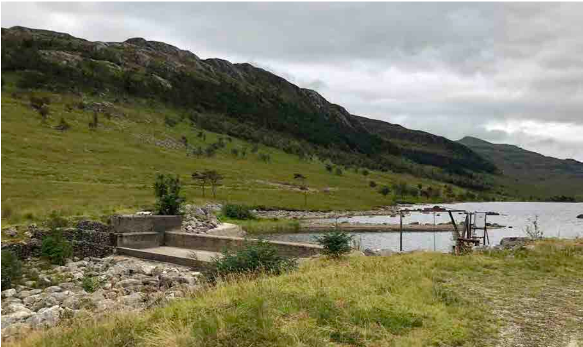
Figure 14 A view of the northern dam from the opposite bank - this is also the location of the Shios Dam
