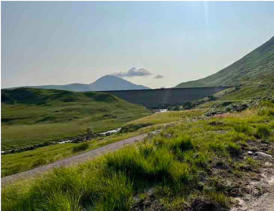
Figure 08 Quoich Dam from downstream
