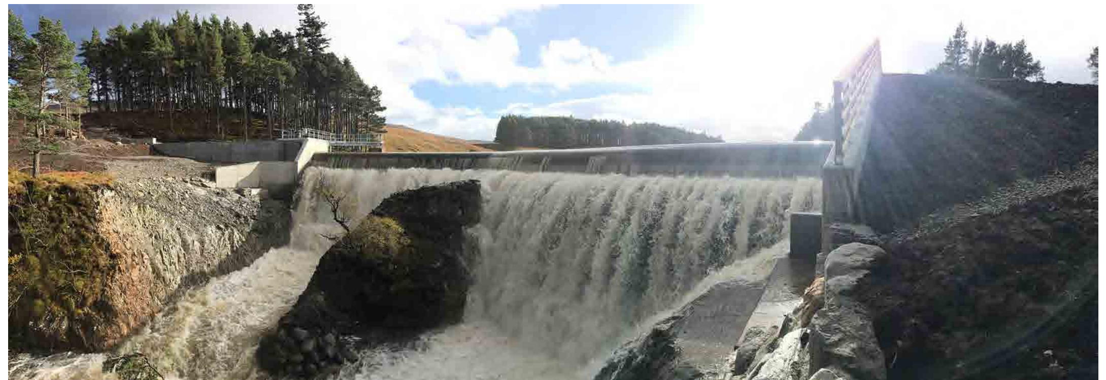
Figure 15 The Pattack Dam
