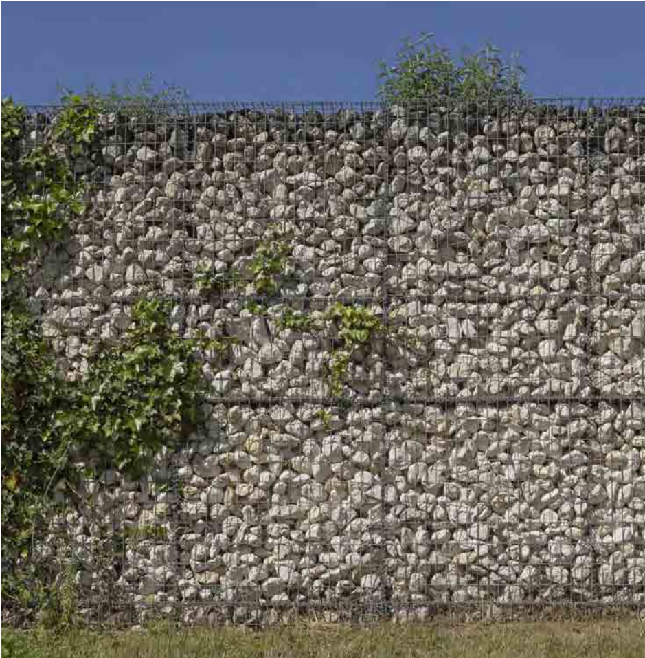
images of gabion construction
