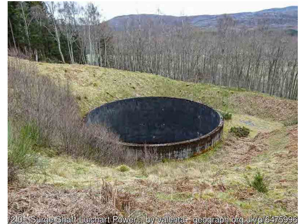
Figure 11 Luichart Surge Shaft with bund surrounding the shaft, but fence placed on the more visible outside of the bund
