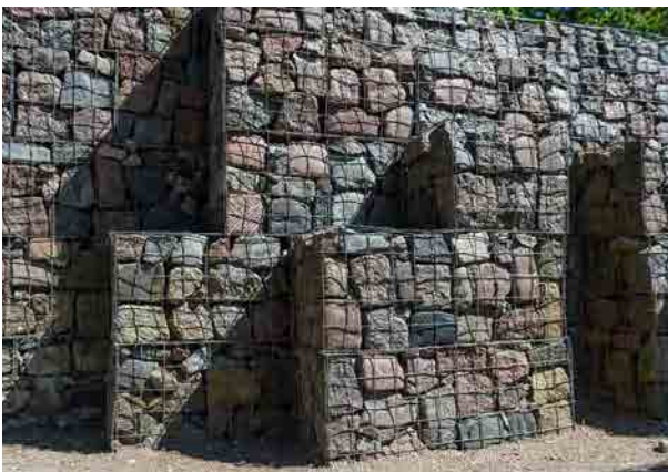
06 - stepping of gabion wall
