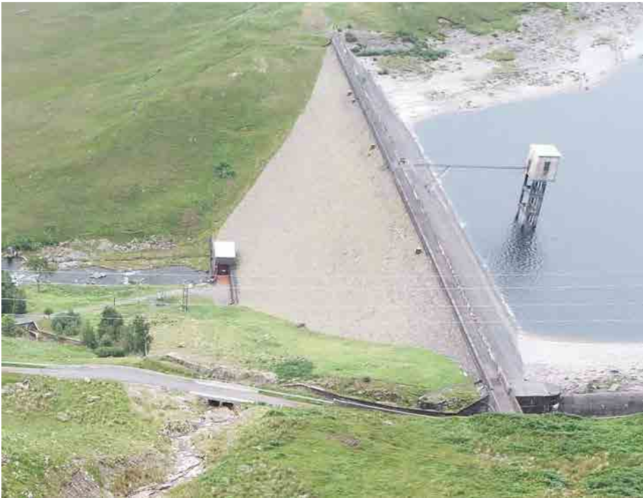
Figure 10 Quoich Dam from above with green mosses visible on dam face
