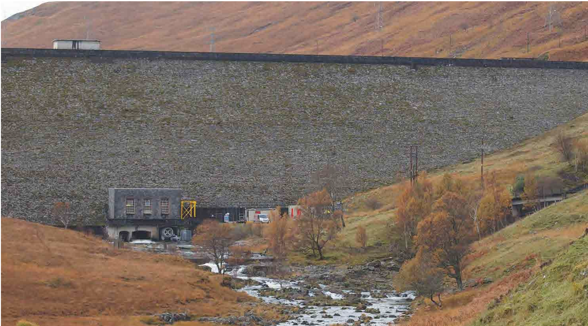
Figure 10A Quoich Dam rockfill elevation, moss establishing on the dam face & intake protruding above the dam
