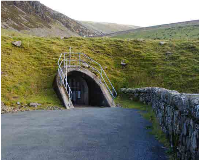
Figure 30 A further Dinorwig tunnel adit
