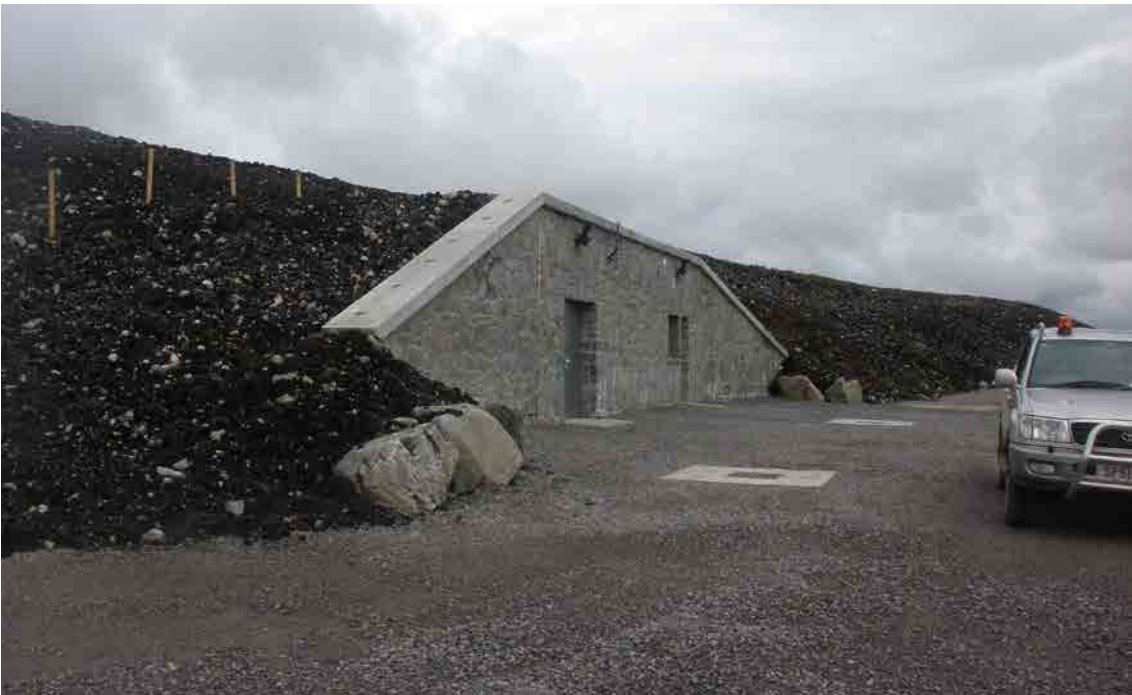
Figure 27 The semi buried Glendoe Welfare building
