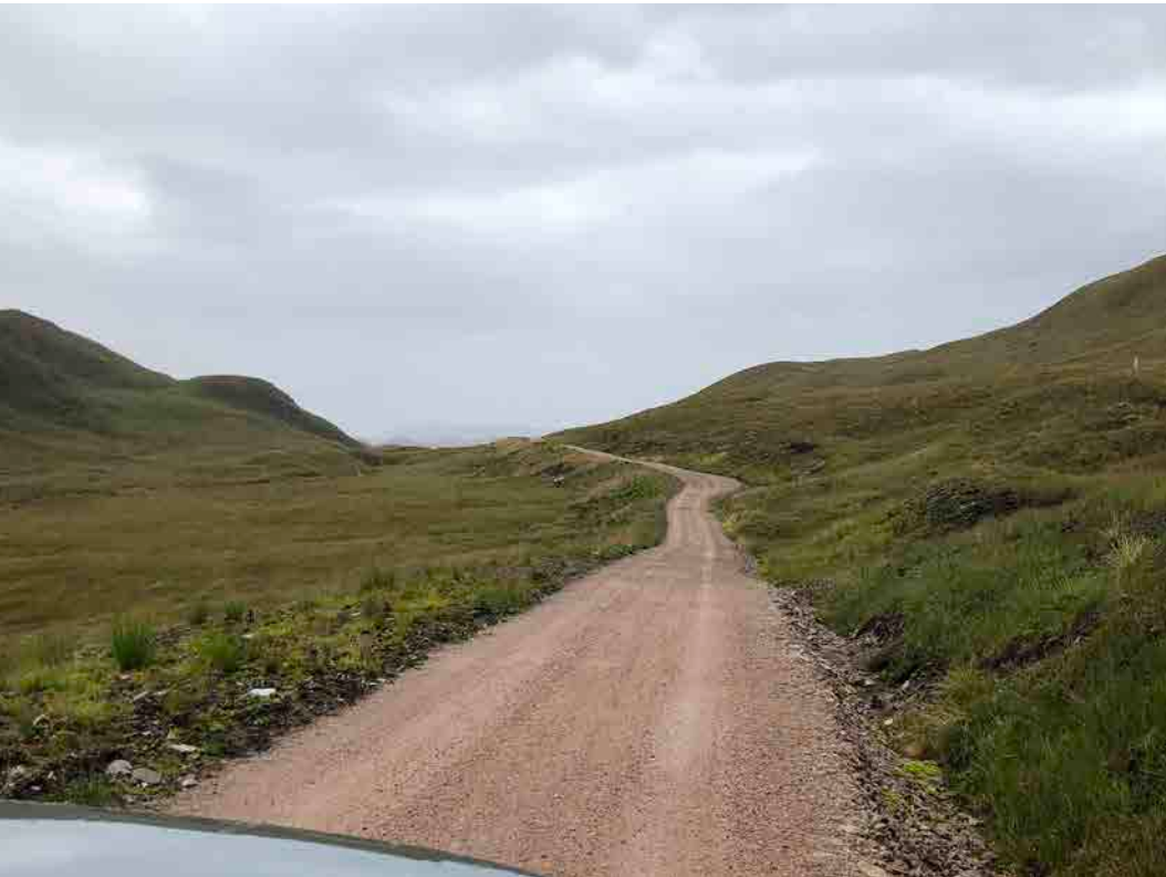
Figure 30A Twin lane construction haul road reinstated to 3m wide
