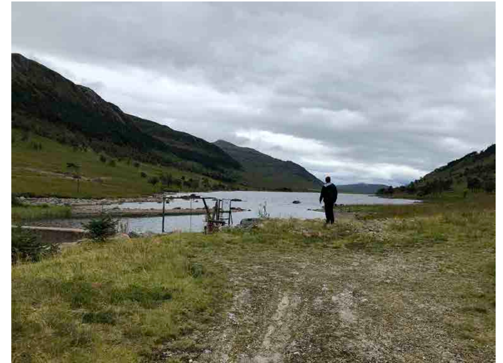
Figure 19 View looking south from Shios Dam, existing intake visible to the left
