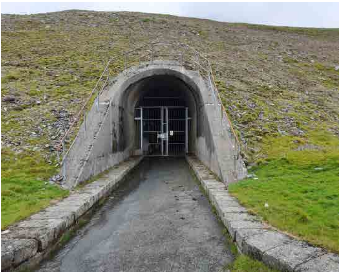
Figure 29 Dinorwig tunnel adit
