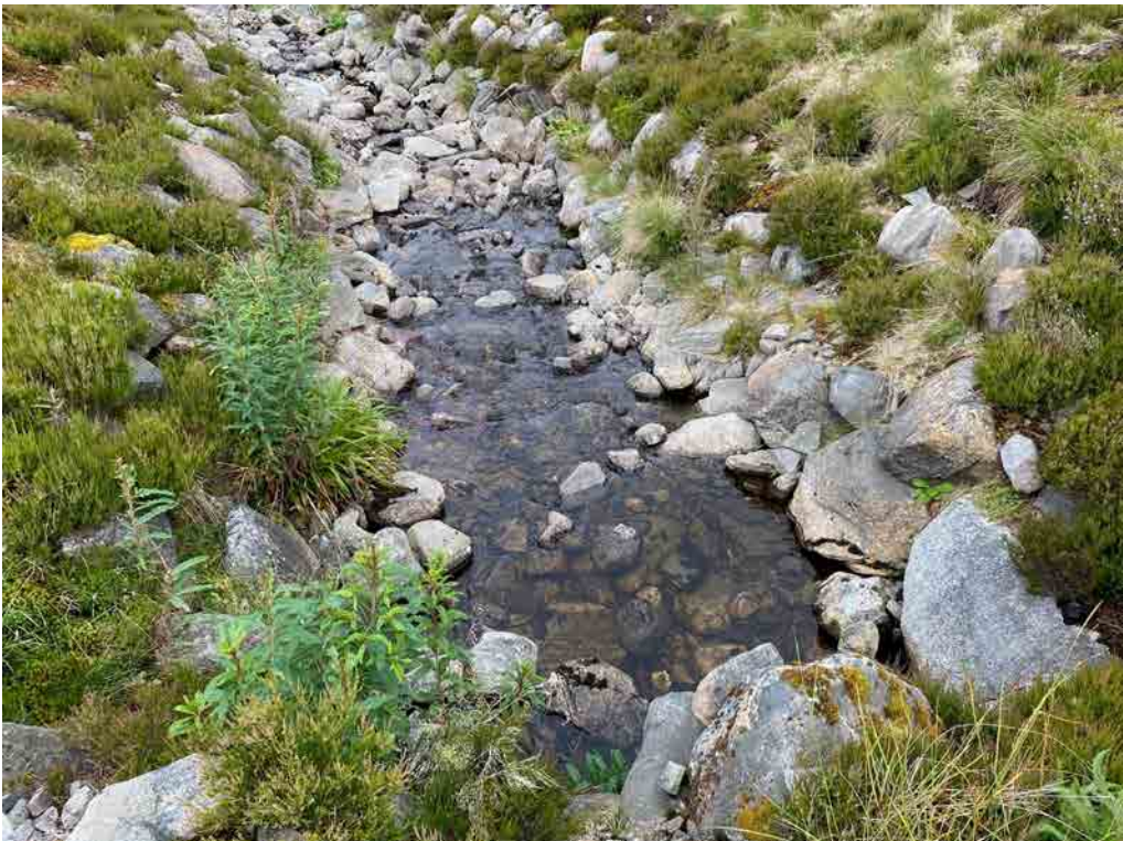
Figure 31 Example channel lined with rock
