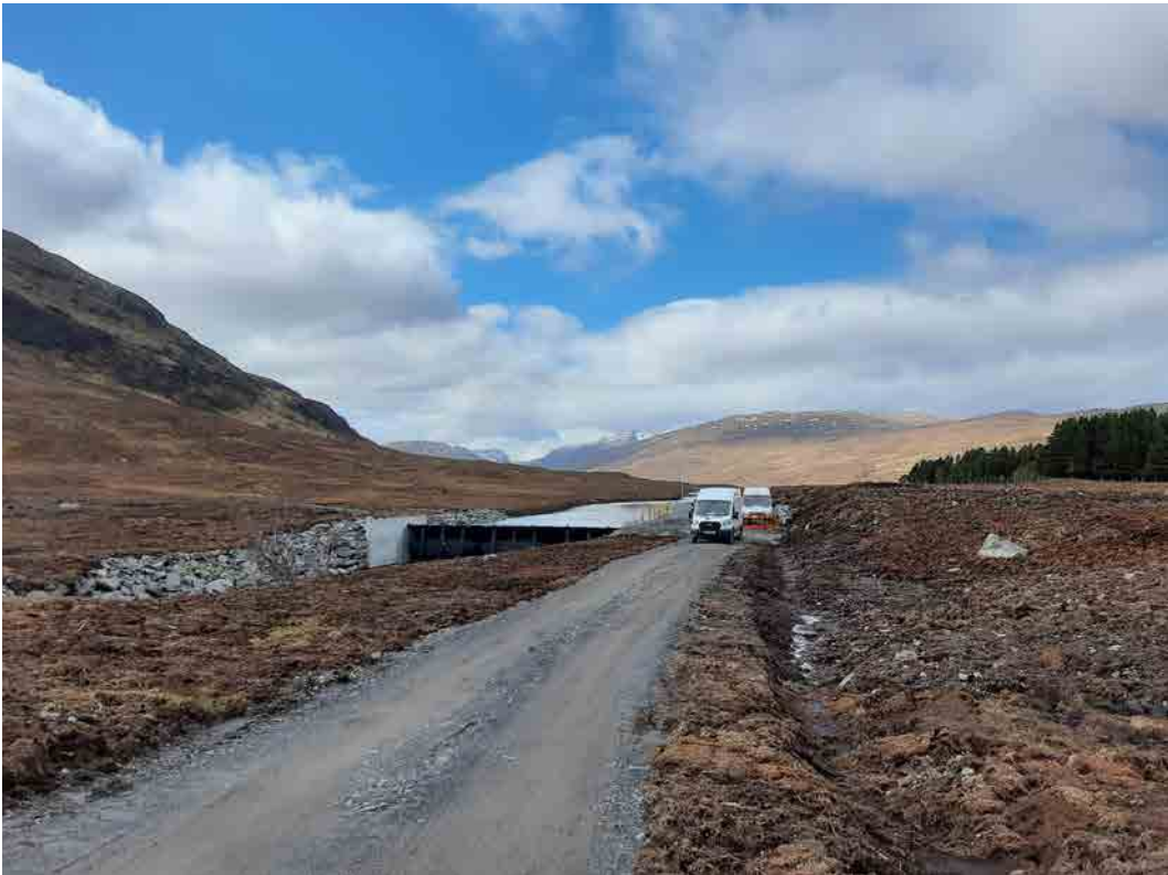
Figure 30B Track to small dam works reduced in scale following completion
