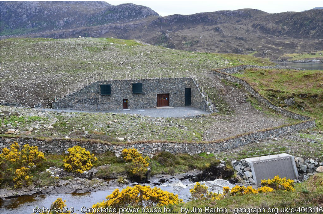
Figure 28 The Maldie powerhouse with only the front face visible
