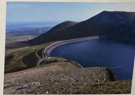
This is Marchlyn Mawr dam in Wales which is similar to the dams proposed at Earba
